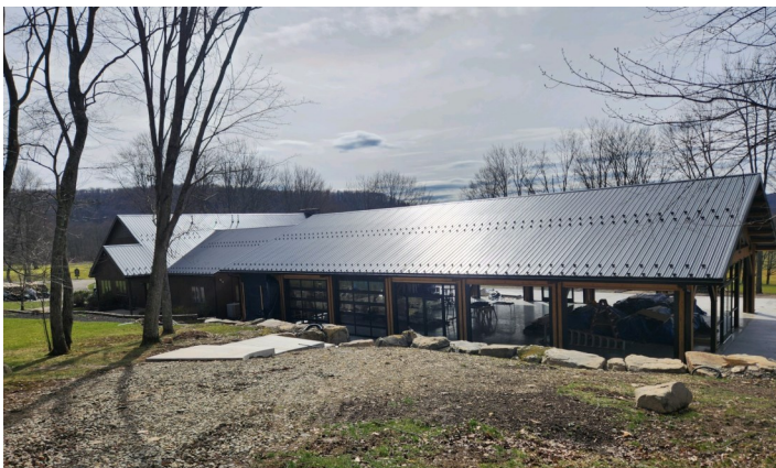
Our gorgeous pavilion is nearing completion!
