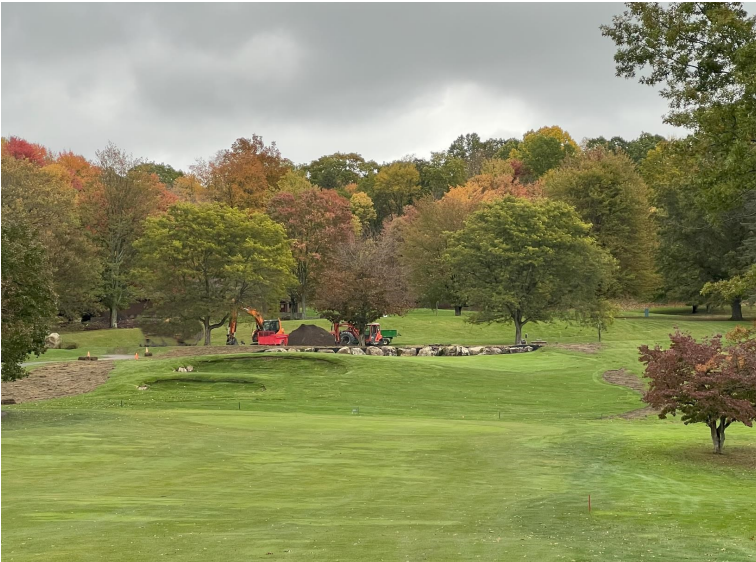
Construction being finished on the new #6.
